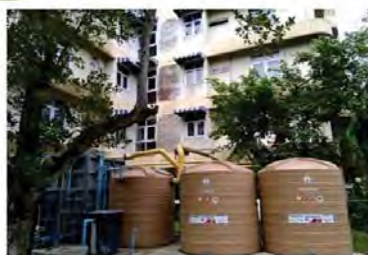
Tanks for recycled water
